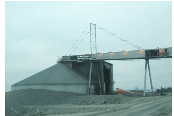
Intermediate storage of primary crushed ore
