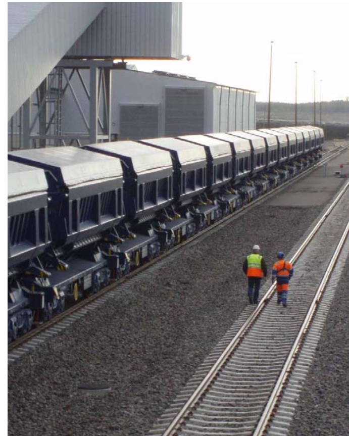
Rail yard at Talvivaara
