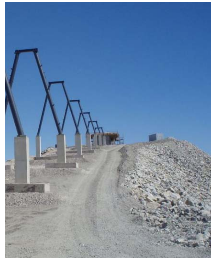
Construction of secondary stacking conveyor line
